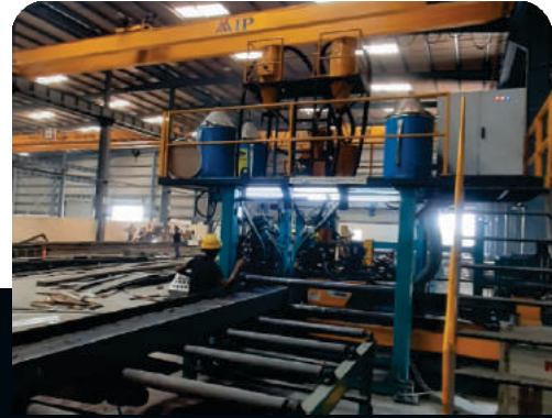
Automatic Beam SAW welding
